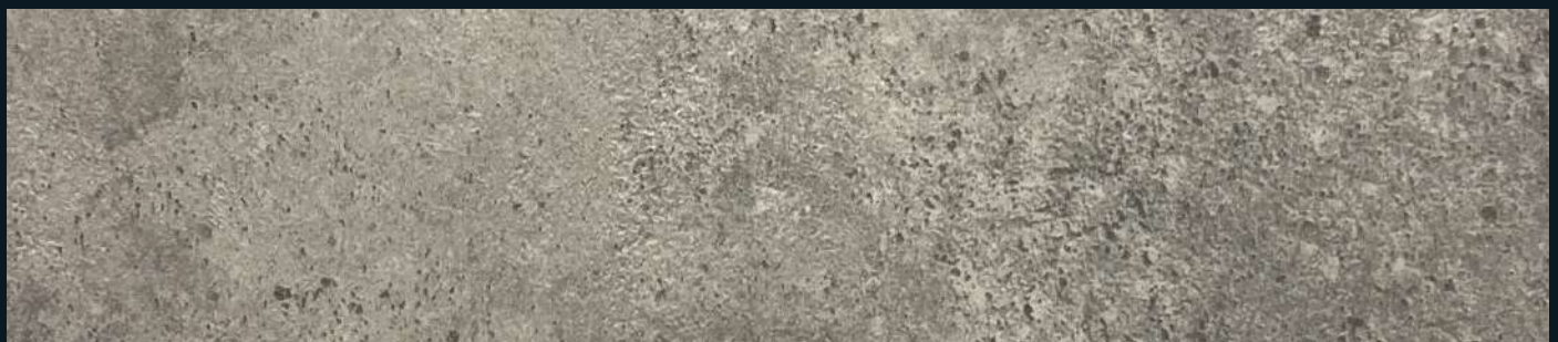
VT SOM23070 / Concrete Dimensions: 4 x 30 m
